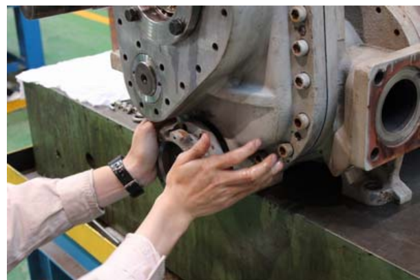
Installing the Unloader Cylinder
