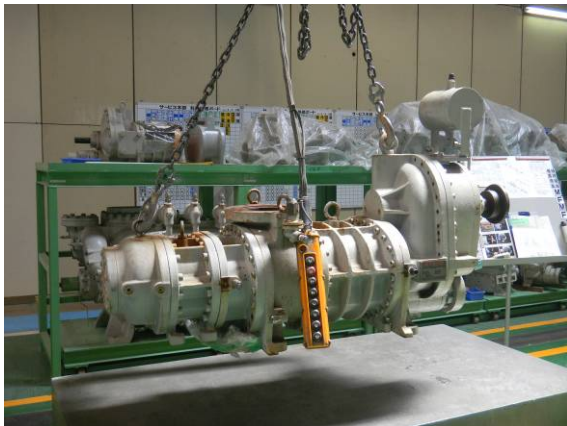
Lifting the Compressor
