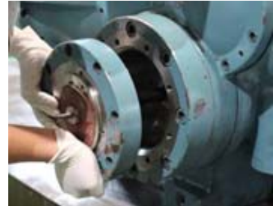
Photo 119 Installing High-stage Unloader Cover
