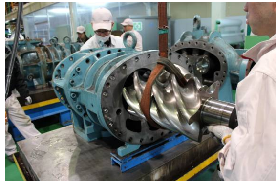
Photo 043 Lifting Up the F Rotor
