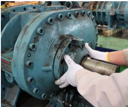
Photo 021: Removing the Seal Cover
