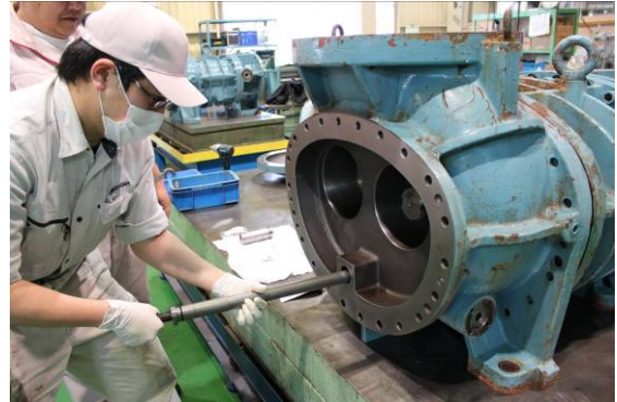
Photo 030 Removing Oil Injection Pipe
