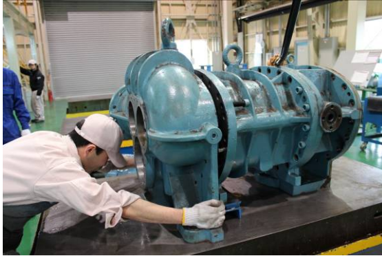
Photo 033 Pulling Out the Suction Cover
