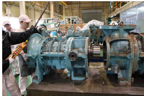
Photo 026: Separating the High-stage and Low-stage Blocks
