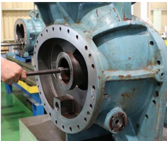
Photo 064 Installing the Low-stage Bearing
